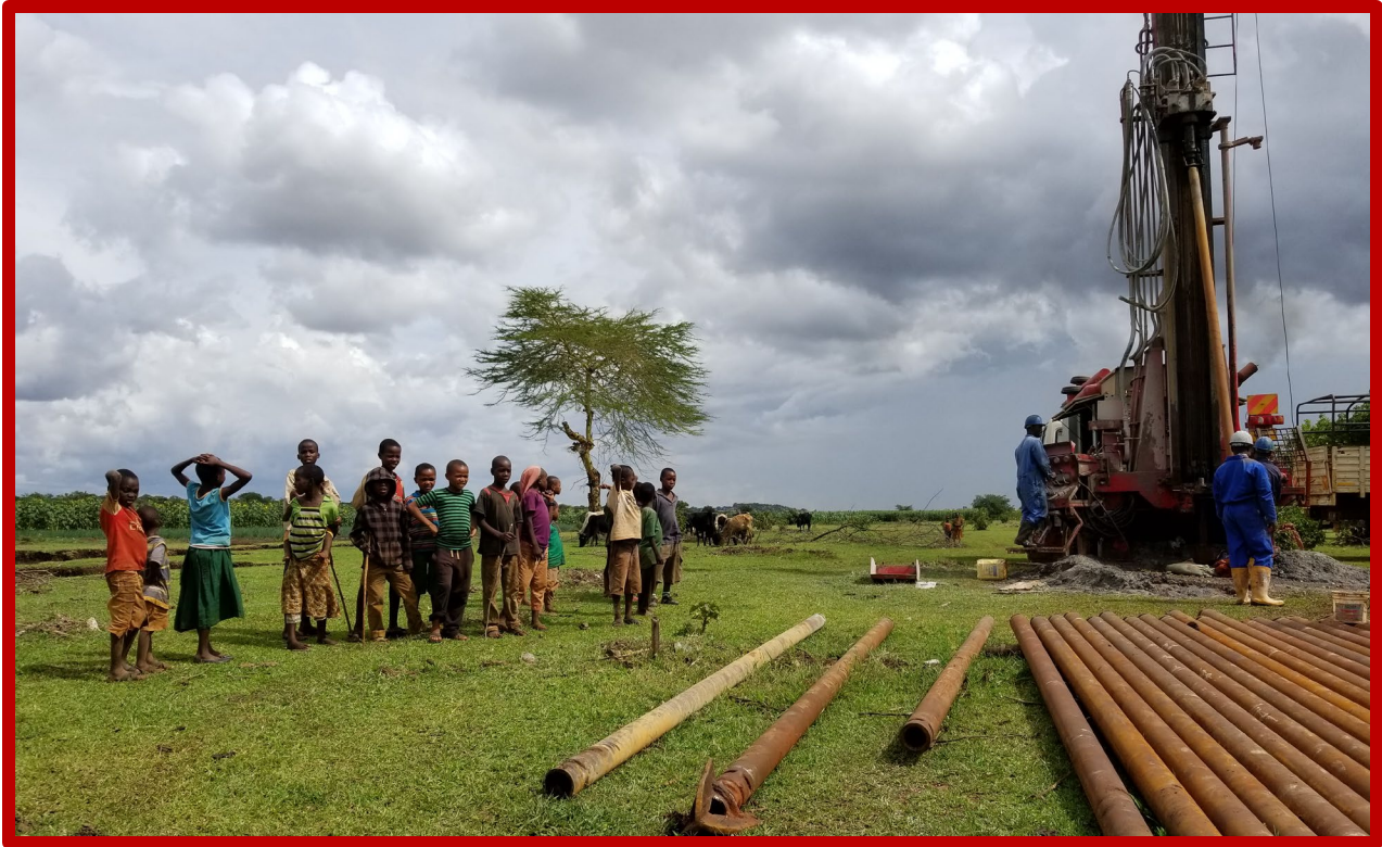
Figure 4: Majitech Engineering drilling a new borehole at Mughanga village, Tanzania, as part of GWI's Sustainable Village Water Systems pilot project in Singida. Image credit: Rebecca Gianotti.
